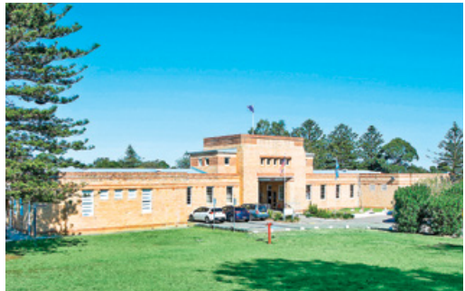
Building 6 (Gate House), North Head Sanctuary. Credit: Mauricio Caicedo.
