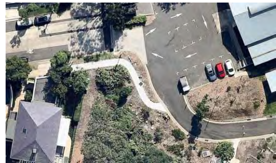
Figure 3.3: Cross Street footpath before upgrades (aerial taken 15 April 2018)
