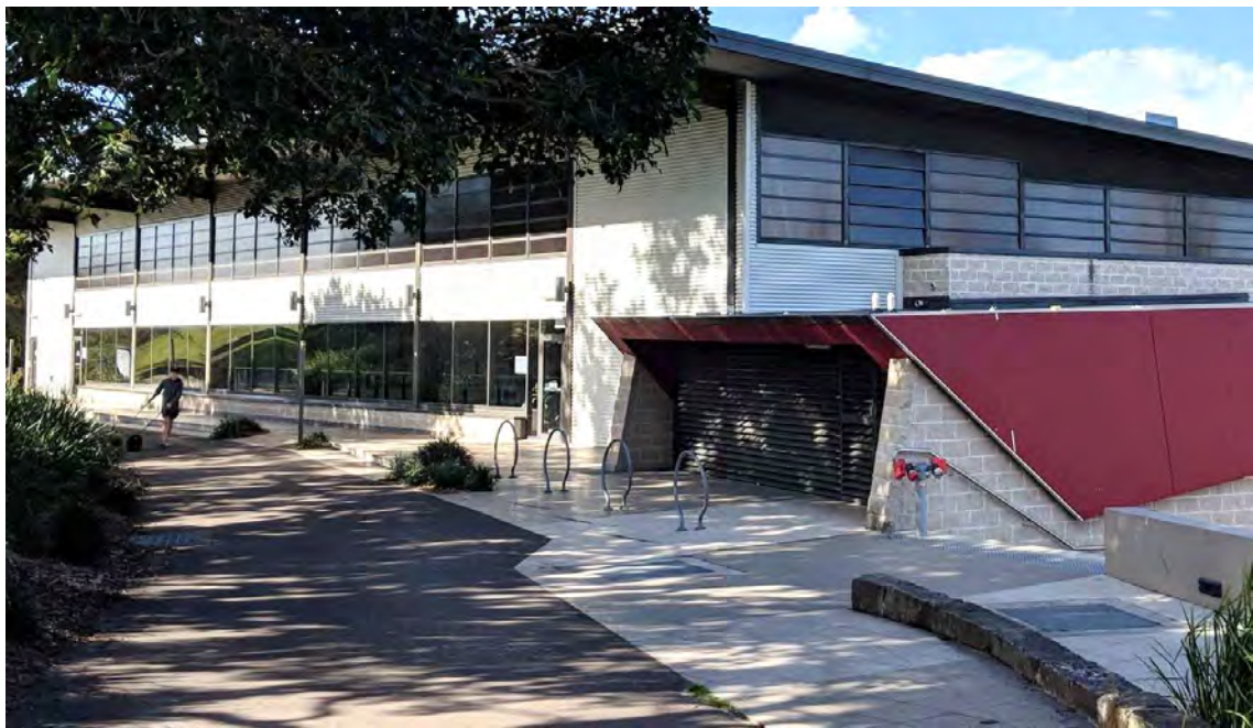
Figure 2.20: Class 3 bicycle racks outside Marie Bashir Mosman Sports Centre
