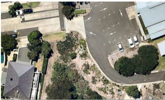
Figure 3.2: Cross Street footpath before upgrades (aerial taken 18 January 2018)
