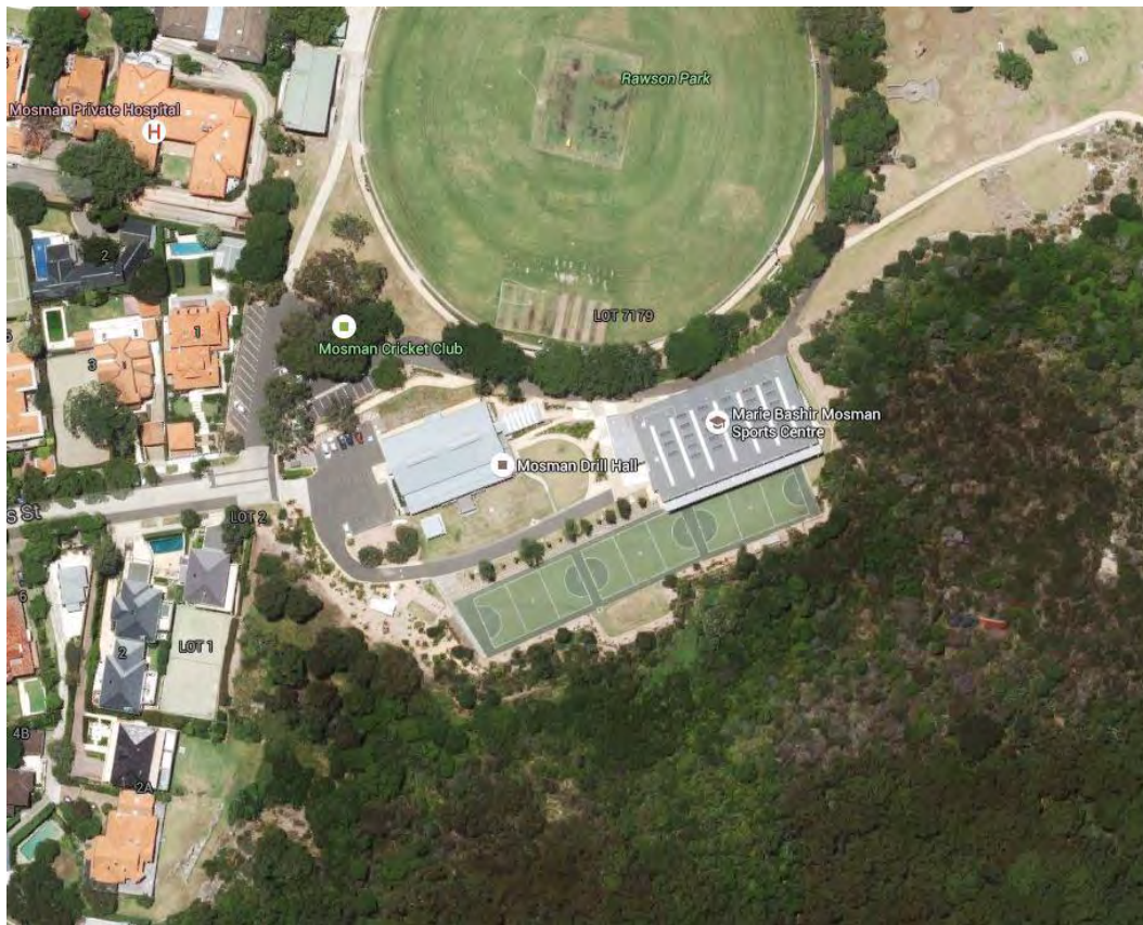
Figure 4-1 – Drill Hall Common
