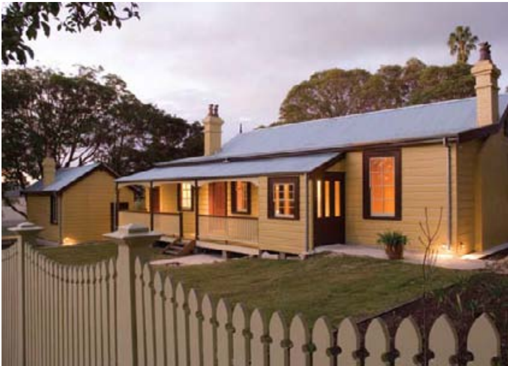
Built in the early 1890s, the Master Gunners' Cottage has been refurbished and is now leased.
