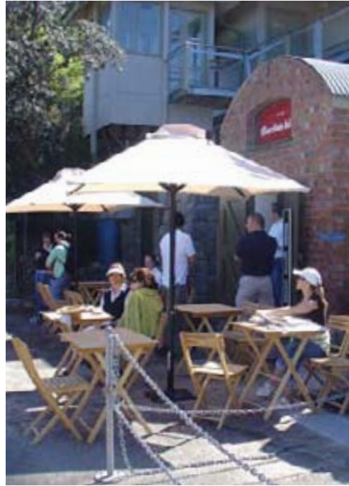
A small brick magazine store, squeezed between sandstone blast walls, used to house explosives, is now a kiosk with an outlook over Chowder Bay and Clifton Gardens.
