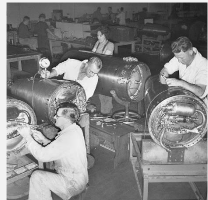
Personnel of the RAN Torpedo Factory overhauling and testing an American Aircraft Torpedo, Unknown, 1945, From the collection of Sydney Harbour Federation Trust
