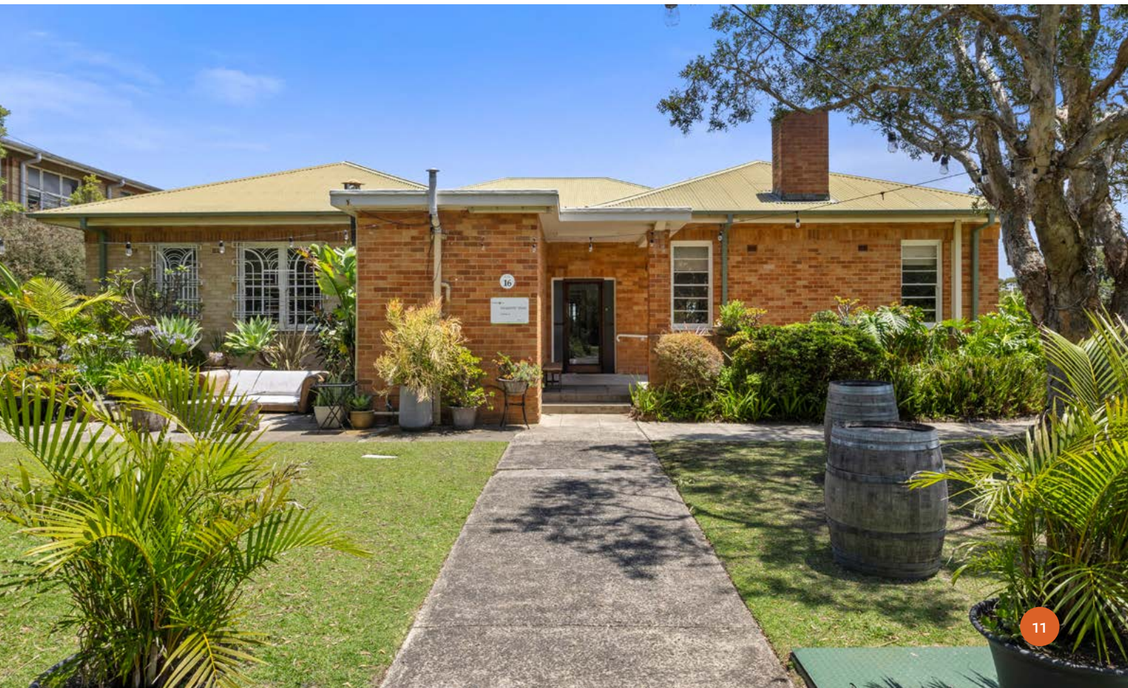
Image: Main entrance, Former Sergeants' Mess, Building 16
