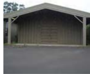
Air Defence Lecture Room & Store c.1956-1962 34A NLA – 144.3m 2
