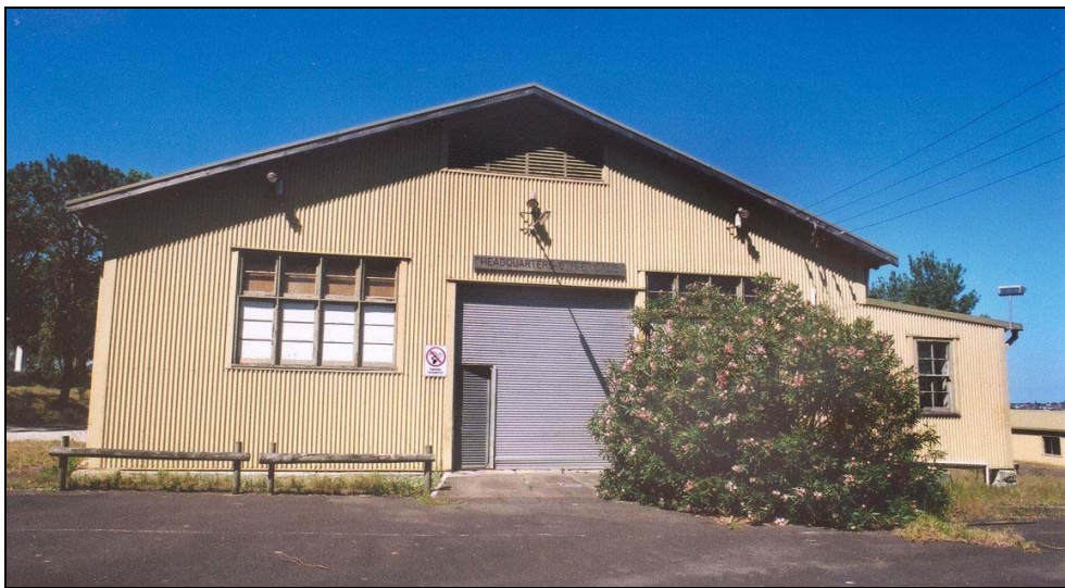
Figure 4: 2002 – Front elevation of the Mosman Drill Hall, with part of the parade ground shown in the foreground. The hall was originally clad with corrugated iron that was fixed horizontally.
