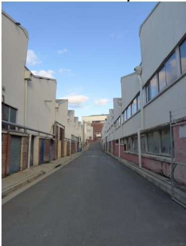
Figure 25: View looking south along the ‘laneway’ between the FIMA Workshop (Building 10 on the left) and the Submarine School (Building 2 on the right).
