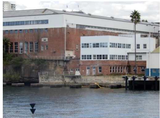
Figure 42: View of RANTME Factor building as seen from Neutral Bay with the RANTME Office building adjacent- proposed location for new Arrival Plaza.
