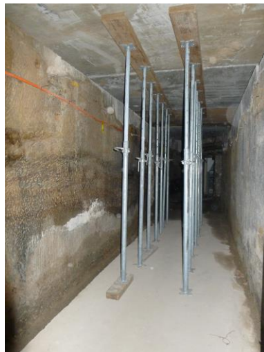
Figure 34: Internal view of the tunnel connecting the Submarine School building to Building 3.
