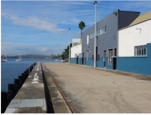
Figure 27: Waterfront façade of Building 10. The larger central section is to be demolished for new courtyard/plaza.
