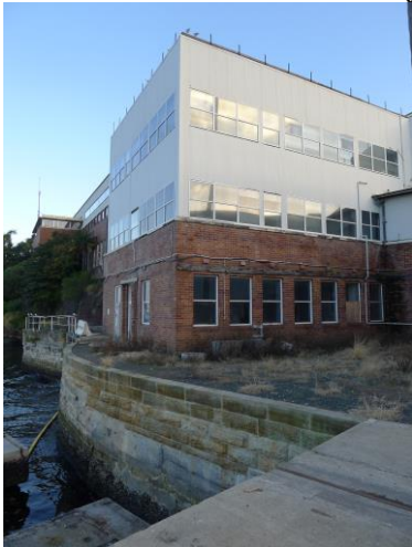
Figure 39: View of RANTME Office (Building 3) to be demolished (not part of this proposal) and new courtyard/plaza introduced on waterfront.
