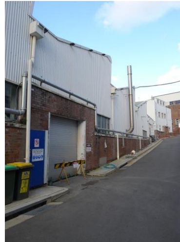
Figure 28: Rear elevation of Building 10 showing bay to be demolished for new courtyard/plaza.
