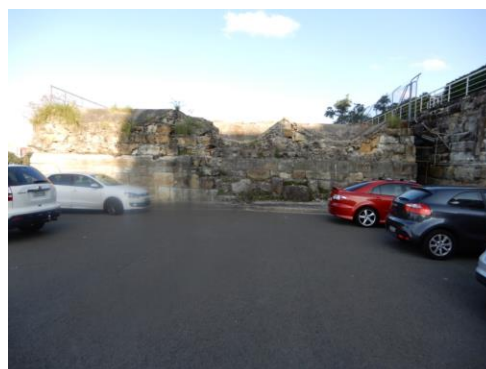
Figure 38: View of Coal Stores from Upper Level Car Park.
