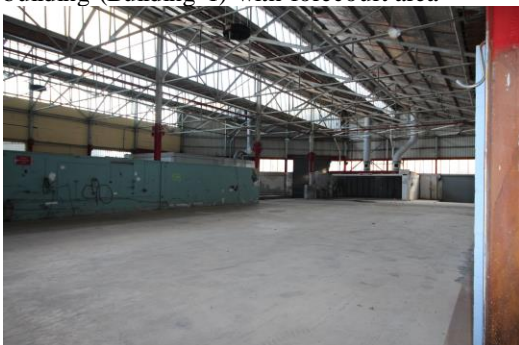
Figure 18: Internal view of RANTME Factory building.
