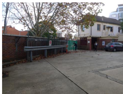
Figure 24: View of forecourt area with Gatehouse in background.
