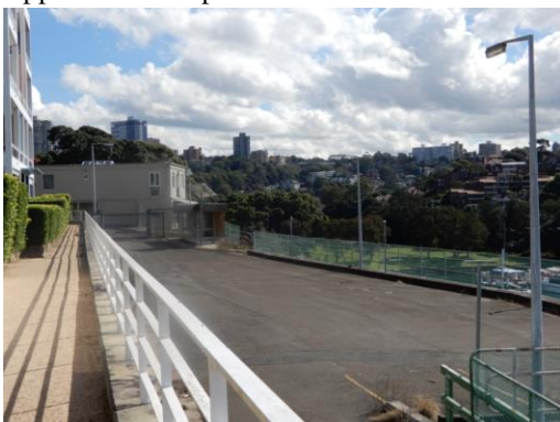
Figure 11: View looking north along length of Upper Level Car Park with Anderson Park in the background.
