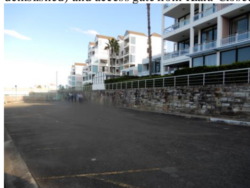
Figure 12: View looking south along length of Upper Level Car Park with the Iora Apartment complex.
