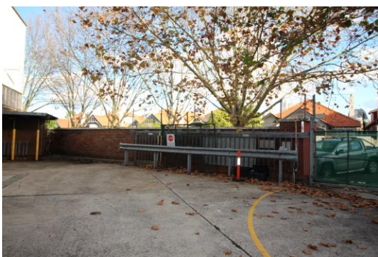
Figure 23: View of front wall to forecourt area
