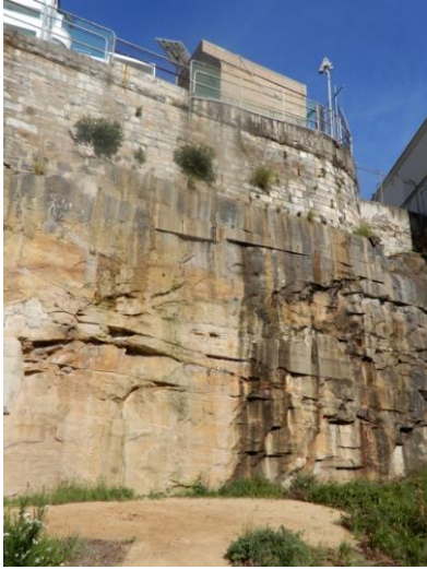
Figure 13: Existing man-made excavated rock face with stone retaining wall above separating the Upper Level and the Waterfront Level of Platypus. The Northern Access Stairway is proposed for this location.
