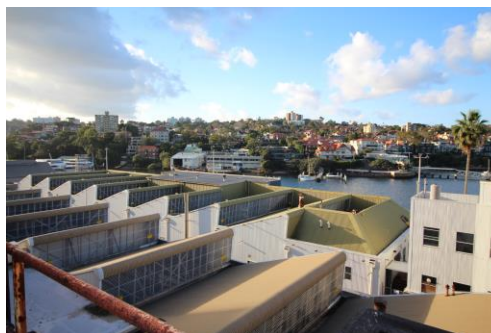
Figure 26: View of sawtooth roofs to Building 2 (foreground) and Building 10 (behind).
