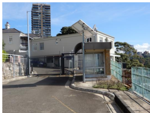
Figure 10: Existing guardhouse (Building 9-to be demolished) and access gate from Kiara Close.
