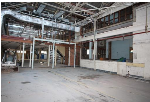
Figure 29: Internal view of FIMA Workshop.
