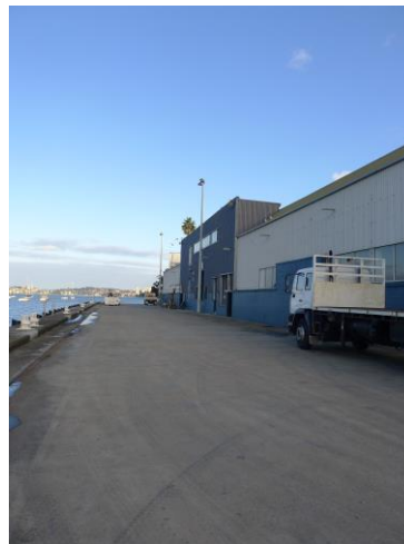
Figure 7: View looking south along the Submarine Wharf with the FIMA Workshop building (Building 10).
