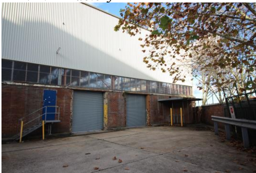
Figure 16: Entry façade to the RANTME Factory building (Building 1) with forecourt area
