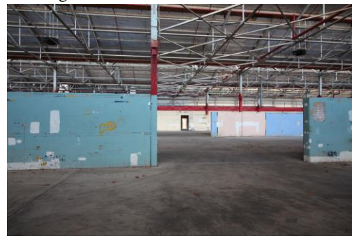
Figure 19: Internal view of RANTME Factory building with blast walls.
