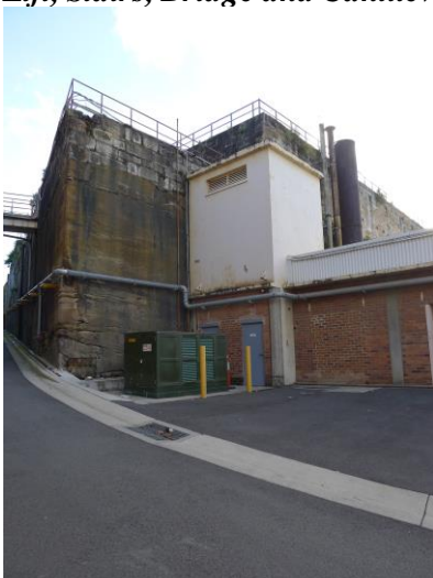
Figure 35: View of southern end of Submarine School building with cliff behind- proposed location of the lift and stairs.
