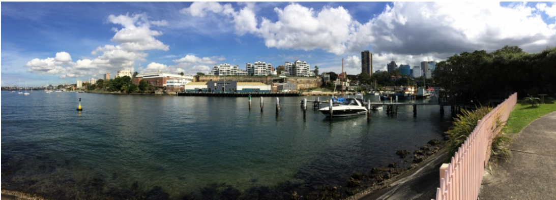
View of HMAS Platypus from the eastern foreshores of Neutral Bay (looking south west)
