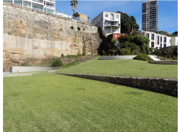
Figure 10: View of the Northern Park and cliff in area where Building 8 was once located.
