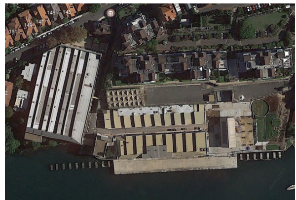
Figure 14: Aerial photograph of Platypus as it is today. Source: GoogleMaps, 2017
