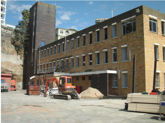
Figure 9: Building 8 with lift shaft once located at the northern end of the site. The lift provided access from the Upper Level Car Park to the Waterfront Level.
