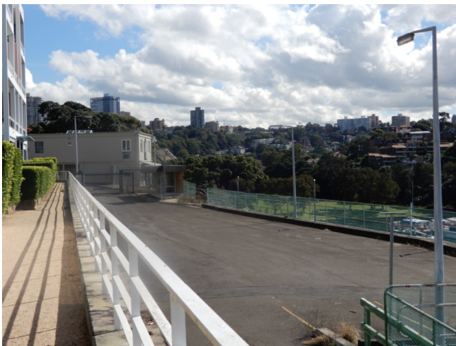
Figure 42: View from walkway in front of the Iora Apartments looking north over the Upper Level Car Park to Anderson Park. No. 9A Kiara Close is seen in the background.
