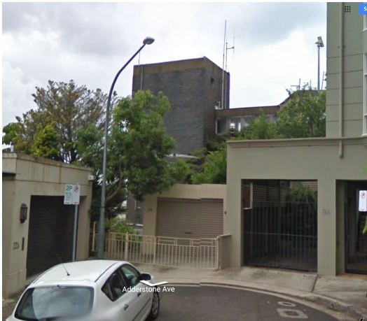
Figure 11: Pre-2012 view from Adderstone Avenue looking south to top of lift shaft for Building 8. Source: SHFT, Google Streetview
