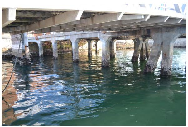
Figure 11 View of wharf support piles and of existing wooded ferry arrester structure inshore from the existing southern pontoon berth.
