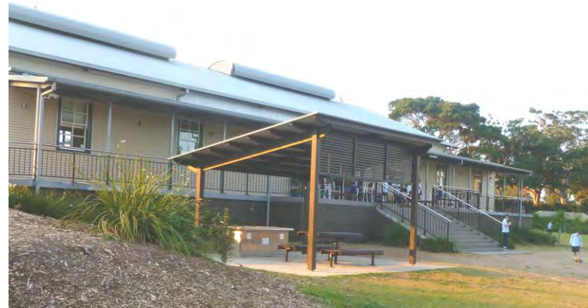
Figure 18: 2018 – South elevation of the Mosman Drill Hall
