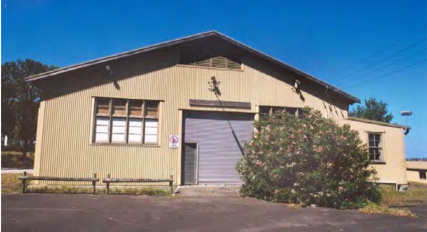
Figure 3: 2002 – Front elevation of the Mosman Drill Hall Part of the former parade ground is shown in the foreground. The hall was originally clad with corrugated iron that was fixed horizontally.
