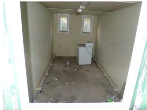
Figure 3. 18: View into former laundry space.
