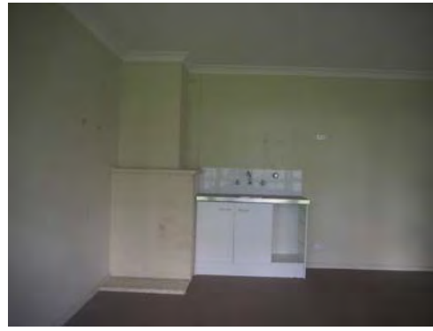
Figure 3. 12: Former common room now partitioned with evidence of original fireplace.
