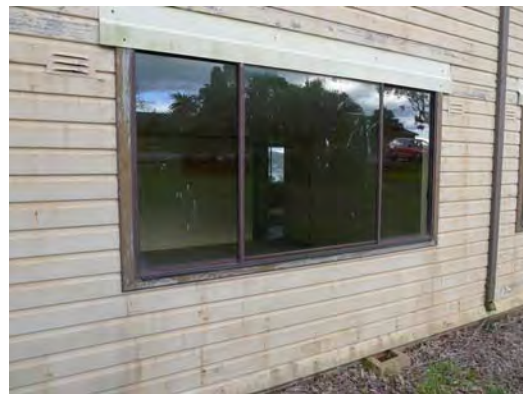
Figure 3. 6: Later addition aluminium framed windows
