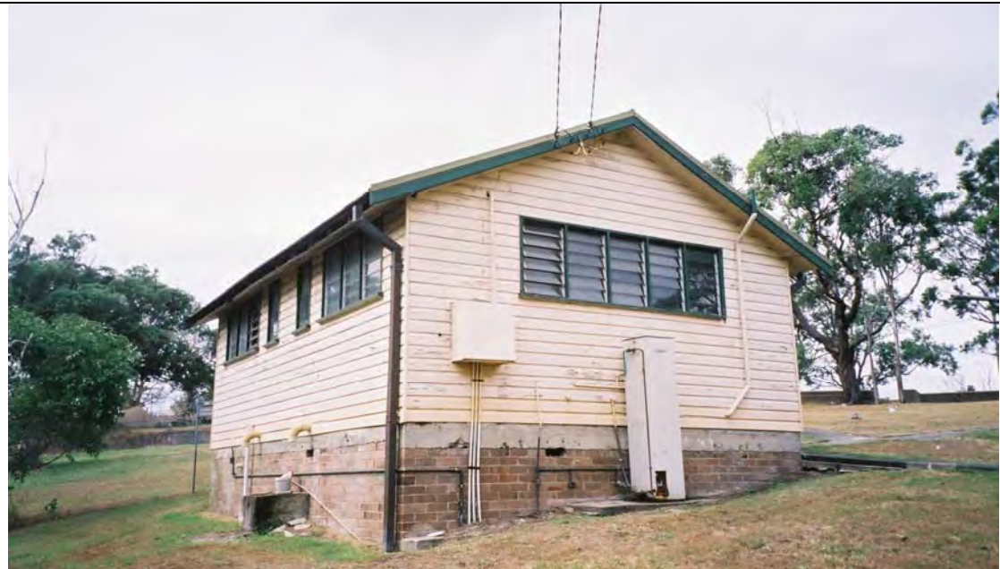
Current view of Building B4 from the north-west (Photo: Robertson & Hindmarsh Pty Ltd, 2006)
