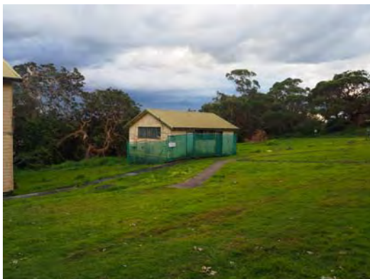
Figure 3. 13: Building B4 in its setting to the east of Building B3
