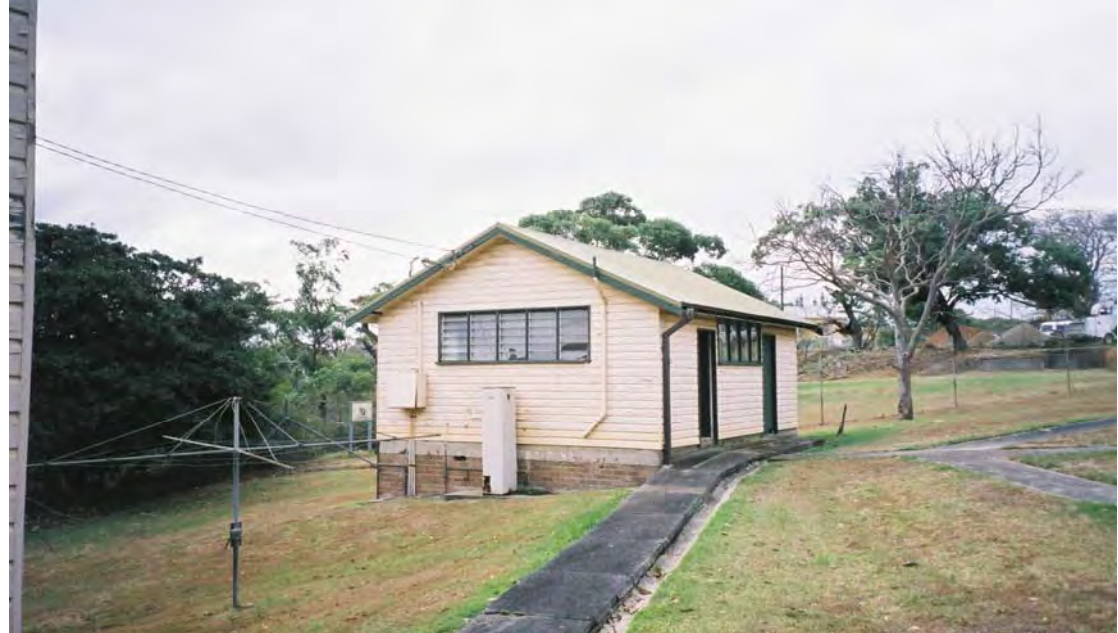
Current view of Building B4 from the south-west (Photo: Robertson & Hindmarsh Pty Ltd, 2006)
