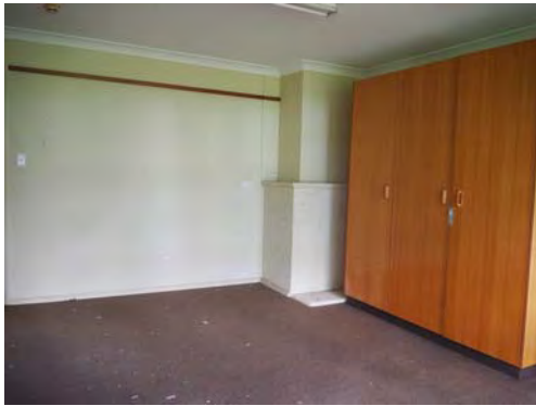
Figure 3. 11: Former common room now partitioned with evidence of original fireplace.
