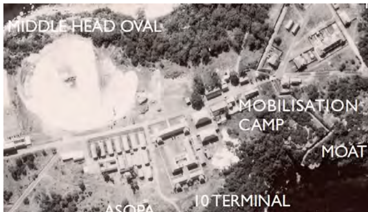
Figure 2. 7: Detail from 1951 aerial photograph of the precinct showing the Anti-Aircraft and Fortress Engineering School and the Signals Camp. By this time the Middle Head oval had been constructed. Source: Middle Head CMP 2007, p. 279
