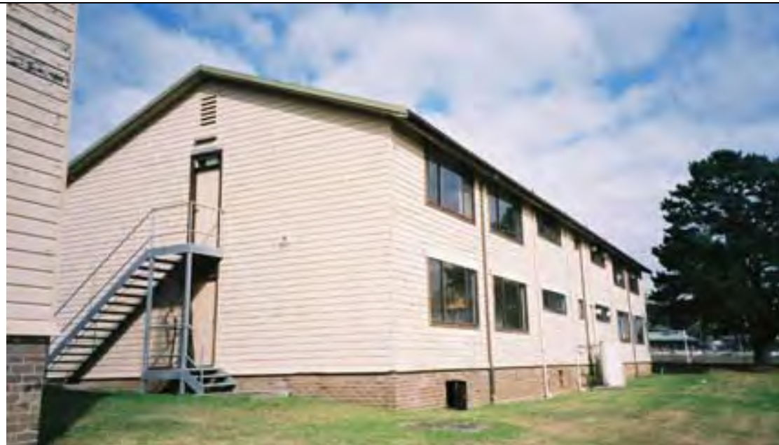
Current view of Building B1 from the north-east (Photo: Robertson & Hindmarsh Pty Ltd, 2006)
