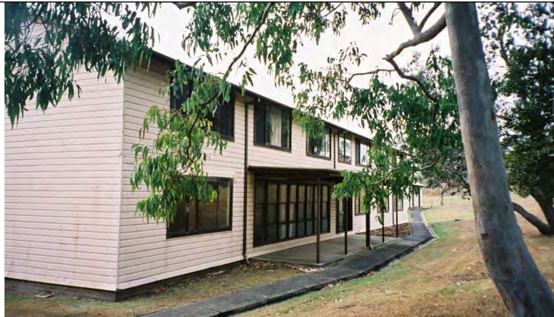
Current view of Building B3 from the south-west (Photo: Robertson & Hindmarsh Pty Ltd, 2006)
