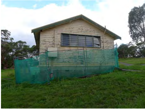
Figure 3. 15: West elevation of Building B4
