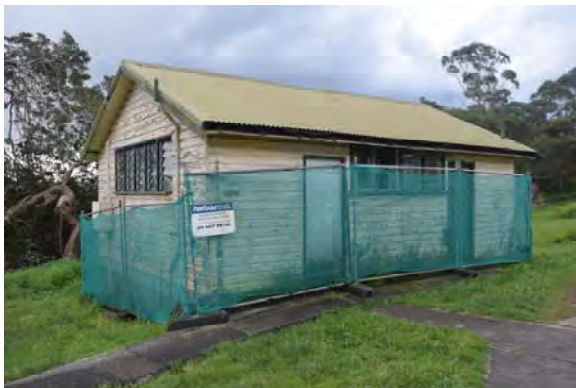
Figure 3. 17: South elevation of Building B4
