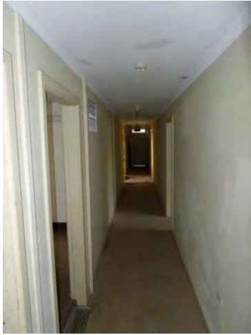
Figure 3. 9: First floor level hallway
