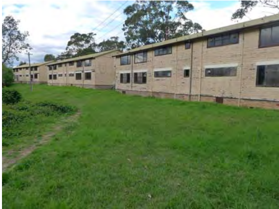
Figure 3. 3: Buildings B1, B2 and B3 (north elevations)
