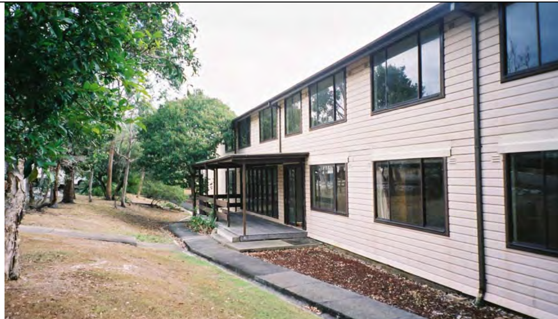
Current view of Building B2 from the south-east (Photo: Robertson & Hindmarsh Pty Ltd, 2006)
