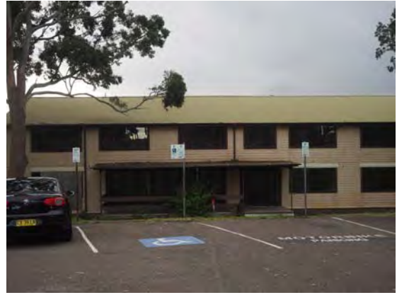
Figure 3. 20: View of Building B2 as seen from the carpark adjacent.
