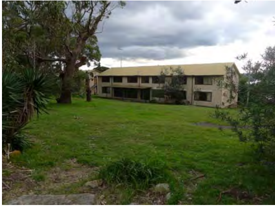
Figure 3. 1: Building B3 (south elevation)
