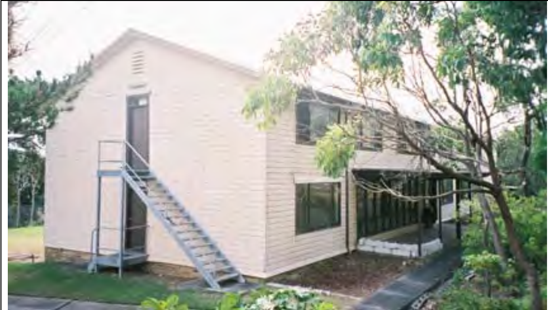
Current view of Building B1 from the south-west (Photo: Robertson & Hindmarsh Pty Ltd, 2006)
