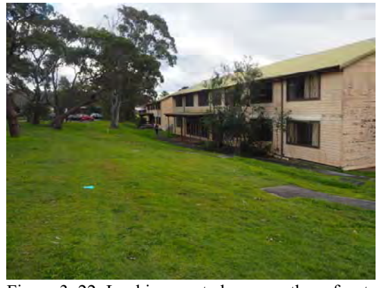
Figure 3. 22: Looking west along southern frontage of the barrack buildings showing the landform
