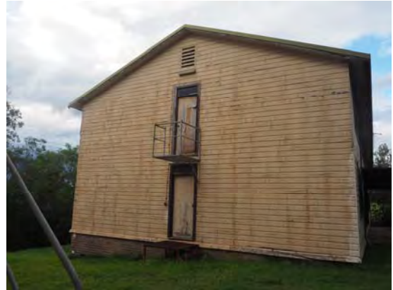
Figure 3. 4: West elevation of Building B3.
