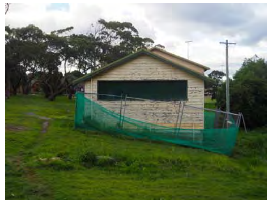
Figure 3. 14: East elevation of Building B4
