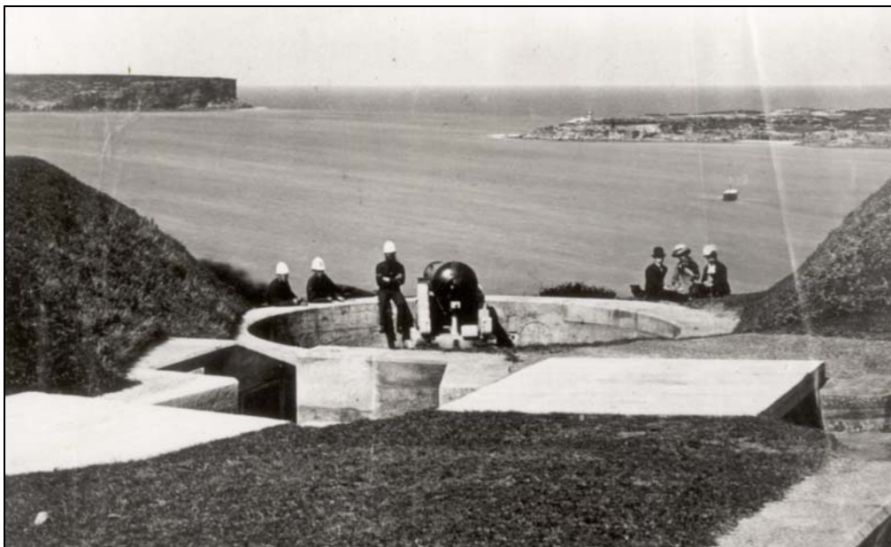
Figure 6: The Georges Head Battery (A84), c.1890. The earth mounds or merlons on either side of the gun emplacements were added to provide additional protection after criticism in an 1877 report that the battery was too open and exposed.
