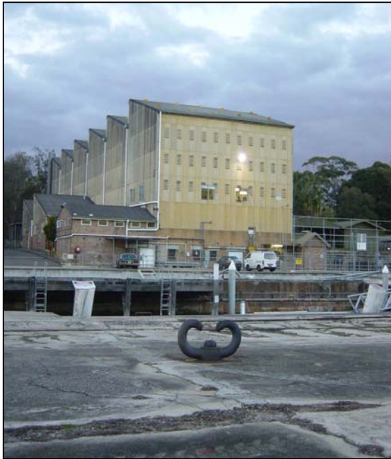
Fig. 18 At the beginning of WW2 Morts replaced many of their small-scale workshops with this impressive saw-tooth roofed building. It is the most significant building surviving from Morts' period of occupation. It is typical of the many industrial buildings which were once common along the foreshores of the upper reaches of the Harbour and the Parramatta River.
