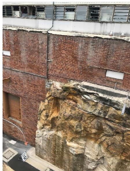
Figure 11: View of line of cut in sandstone base the factory building sits on.
