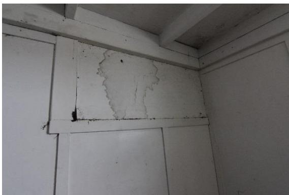
**Photograph 8.43 Evidence of water damage to a portion of internal walling (ERM, 2018)**
