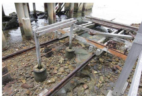
**Photograph 8.32 Iron boat ramp, with heavy corrosion (ERM, 2018)**
