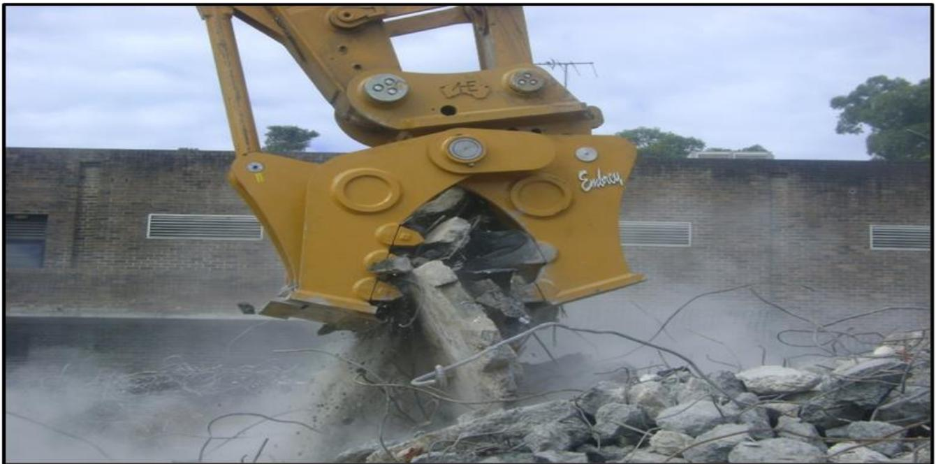
*Figure 4 – Processing of Concrete Materials with Pulverizer Attachment*
