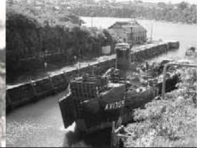
Army landing craft in Woolwich Dock
